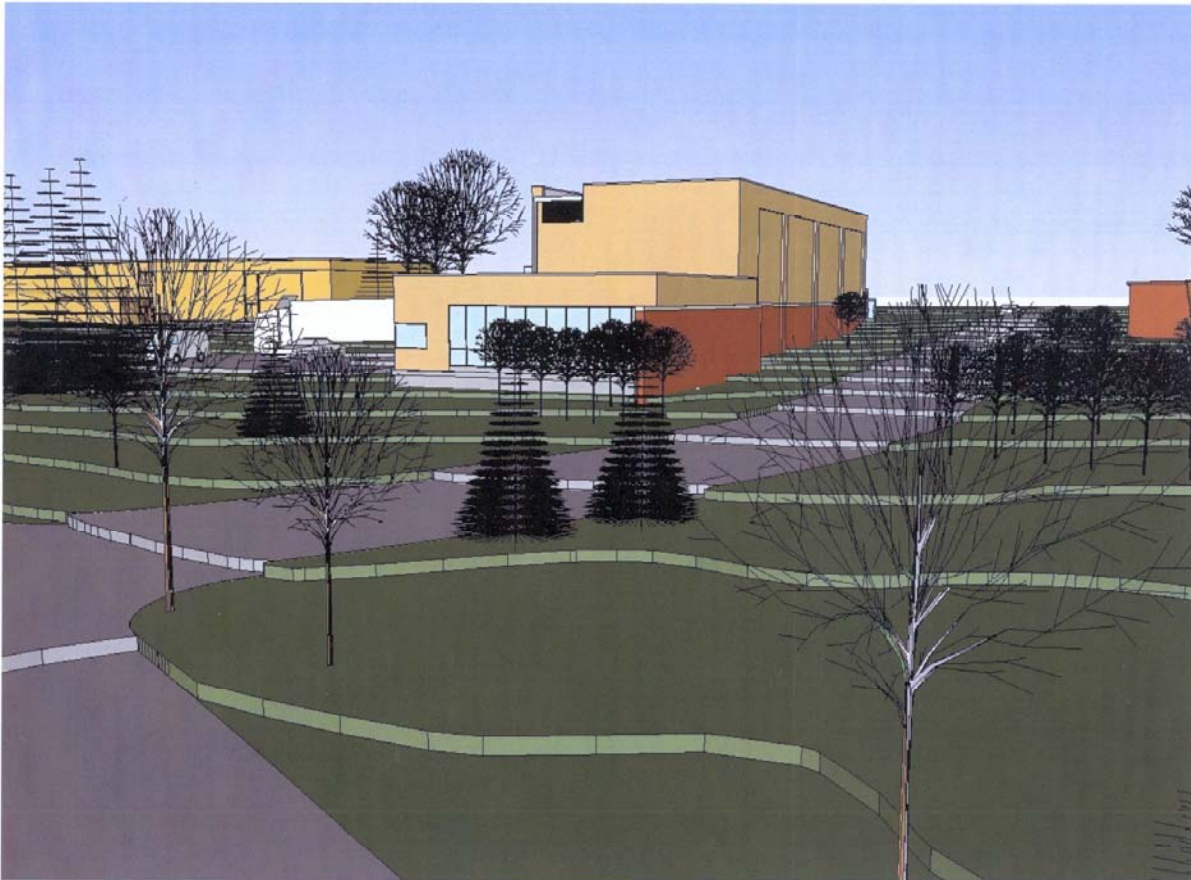
GROUND VIEW LOOKING SOUTH EAST
