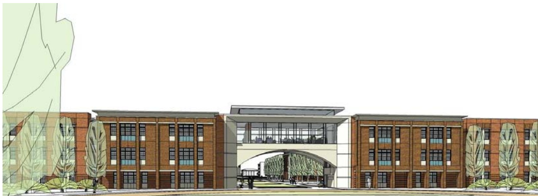
View from 9 th Ave. Campus Edge Looking West
