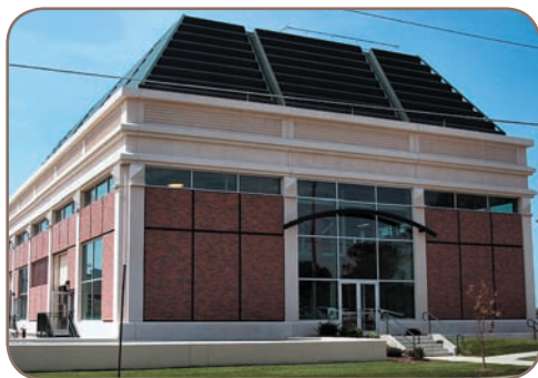
UNMC East Utility Plant
