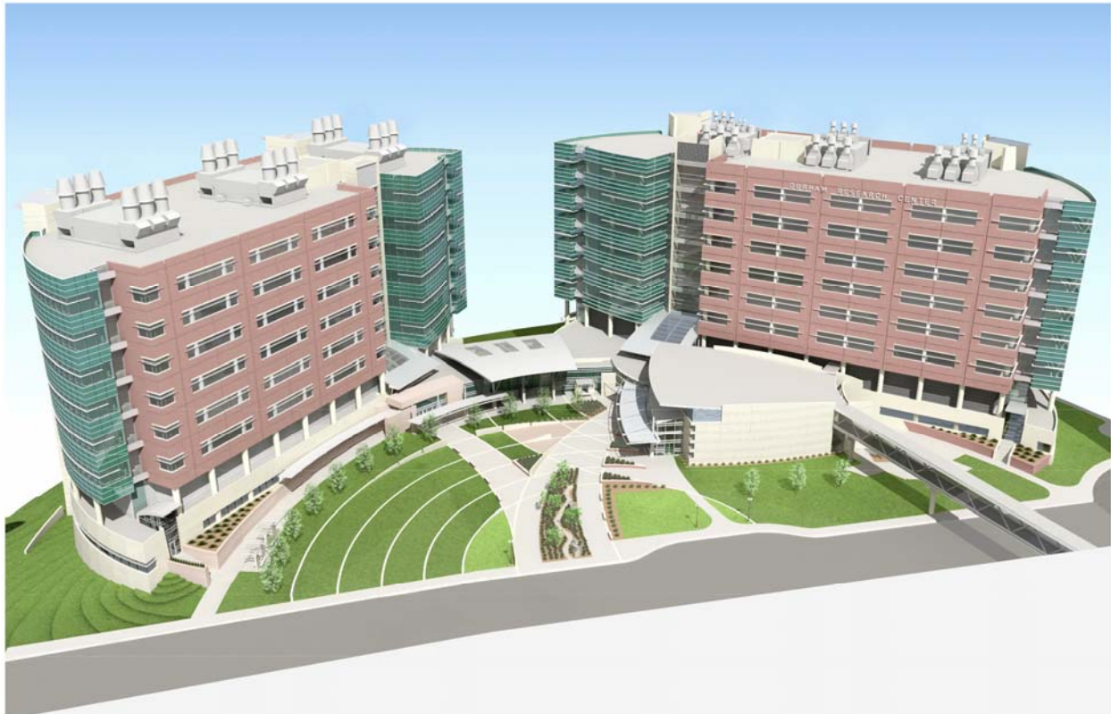
UNMC Research Center of Excellence II East Elevation (Showing the adjacent Durham Research Center on the right)
